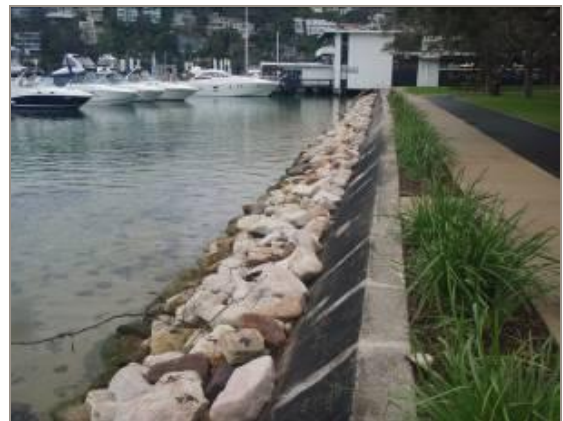
Figure 3. (left) Seawall prior enhancement (right) Rock rubble - artificial reef habitat
