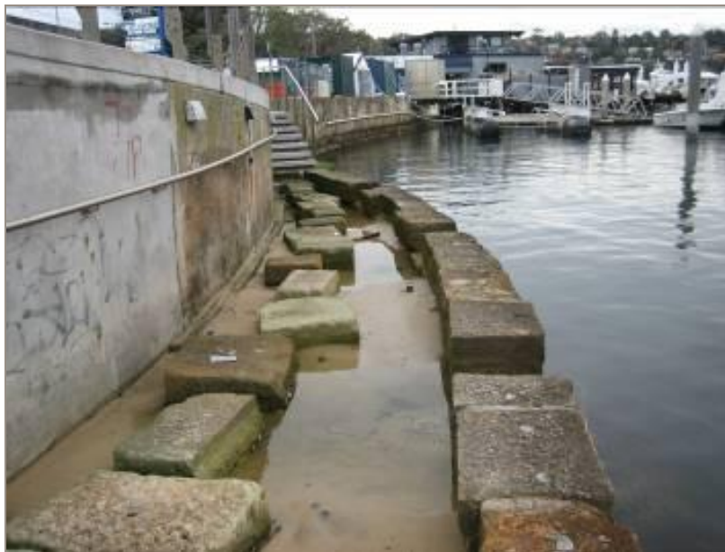
Figure 5. Rock pool created to retain water at low tide
