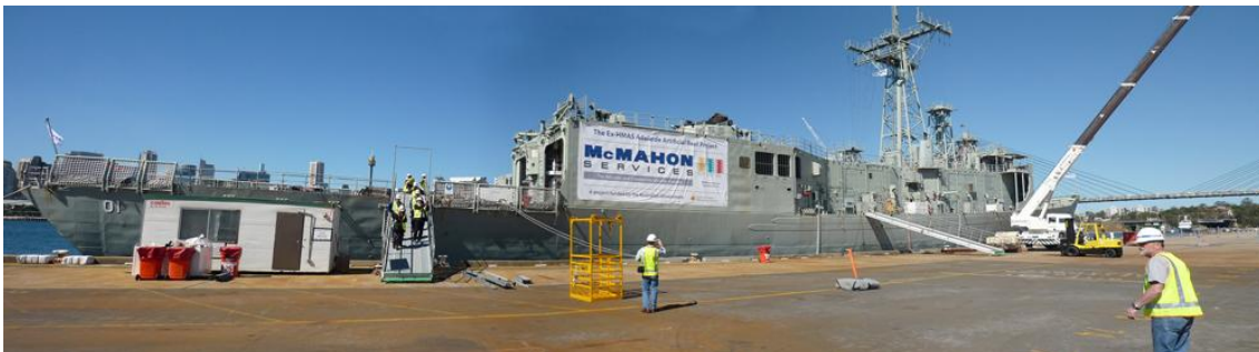
Figure 5: The ship being prepared at Glebe Island Wharf
