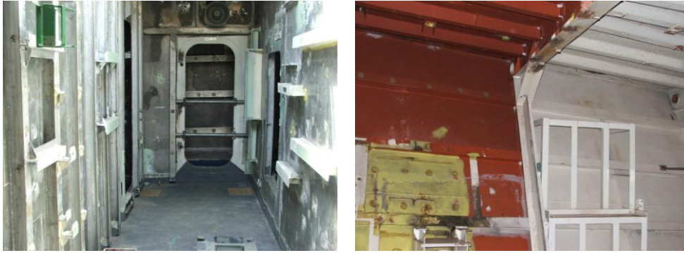
Figure 6: The underlying surfaces after removal of insulation
