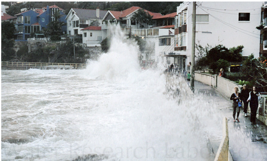
Plate 4. Wave overtopping Fairy Bower, June 2003.
