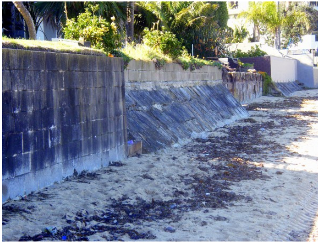
Plate 2. . Seawalls along Clontarf Beach, Sydney Harbour
